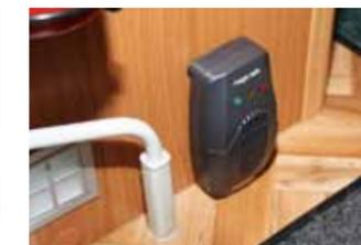
A hard-wired gas detector is part of the system's comprehensive armoury
