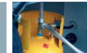
Connect the filler hose to the cylinder filler valve and securely fasten. To turn your system into a twin cylinder system you require a Cylinder-2 and Stainless Steel Connection Hose.
