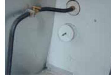
Mark out and cut a 70mm hole for the filler point
