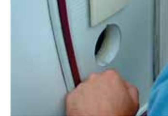
Using a file, create 2 small cutouts top and bottom for the lugs on the filler bracket.
